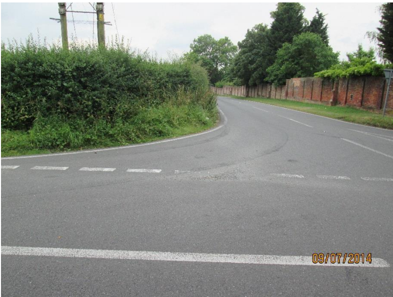
Image 1 – Give-way line proposed left of this position where vegetation will obstruct visibility to northbound vehicles.
